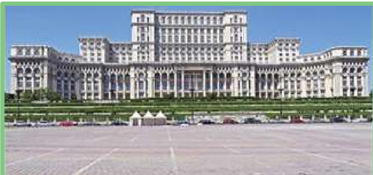
Fig. 4. The front of People's House
