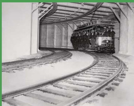
Fig. 2. Tremont Street Subway
